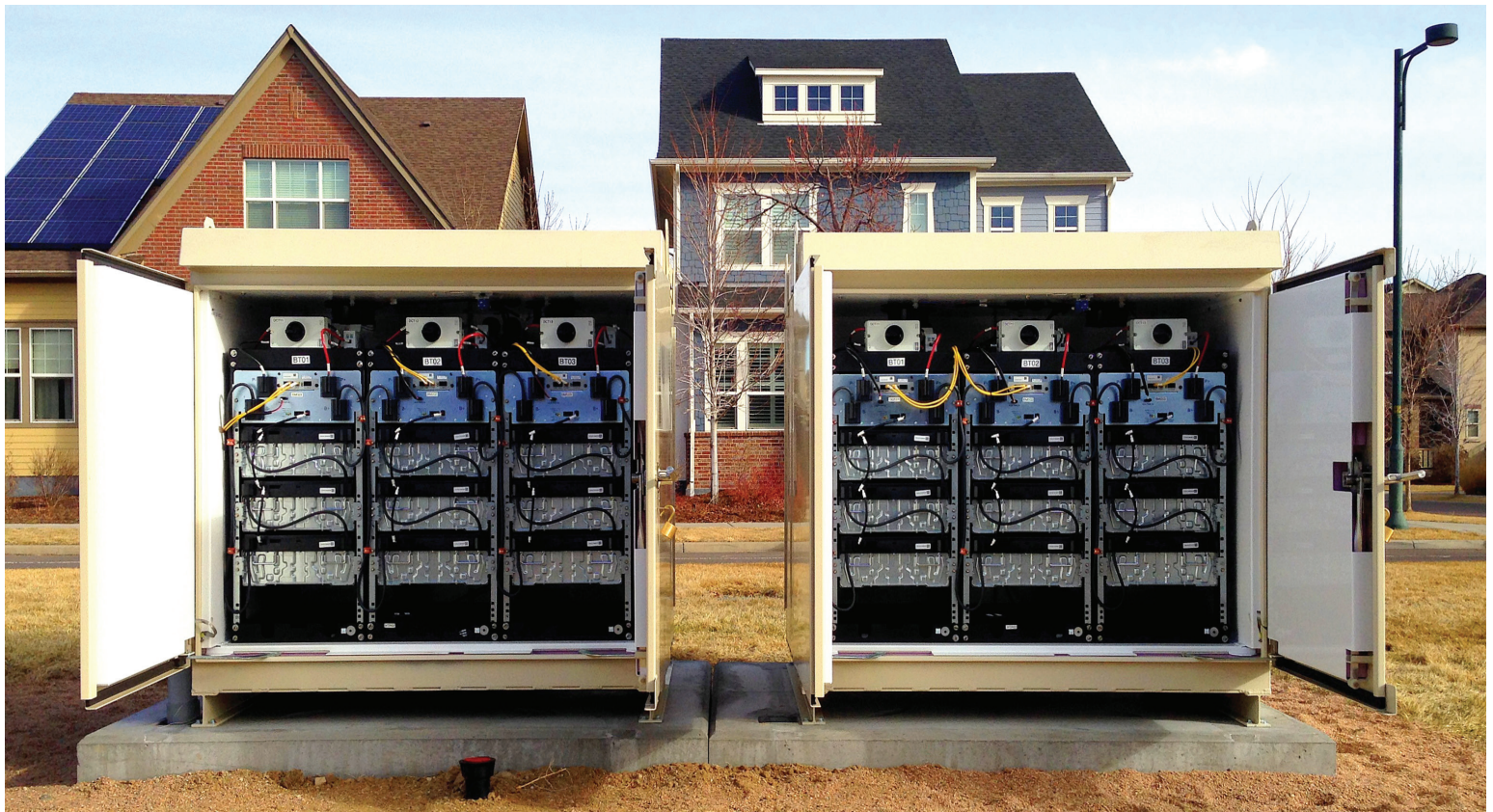
36kW/138kWh AC Storage System (2, side-by-side 18kW/69kWh units)
