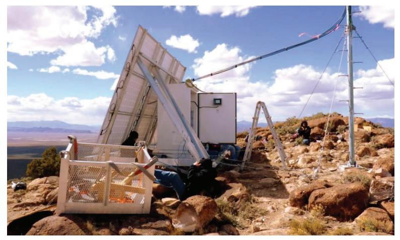
"NRI's solution was a stand-alone solar power system employing a 2.3kW photovoltaic array and back-up generator to charge the battery bank and power the customer loads." - Cubic Operation Team
